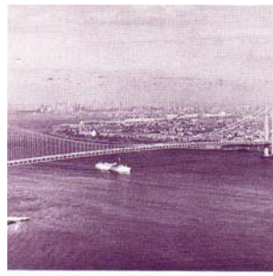
Verrazano-Narrows Bridge linking Brooklyn and Staten Island, New York
